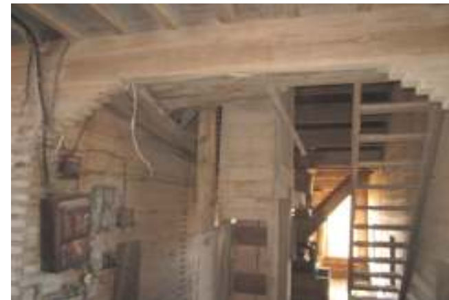
Looking into the main part of the building.
